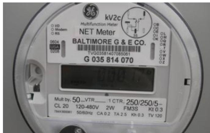
This digital meter runs in both directions to accommodate electricity generated at this customer's home. A 4 kilowatt PV system on a home in this area would offset around 4911 kilowatt hours of electricity each calendar year, saving the homeowner over \$380 on their utility bill. (Source – NREL PV Watts, EIA)
